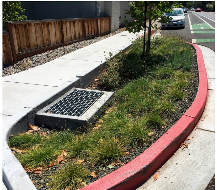
Green infrastructure in Brisbane and the City of Burlingame for neighborhood-scale stormwater capture and diversion (Left: City of Brisbane, Above: Matthew Fabry)
