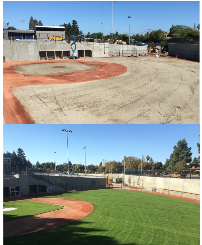
McKelvey Ball Park stormwater detention basin in Mountain View, during and after construction
