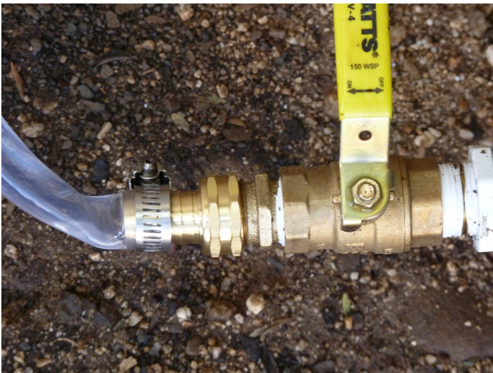
Rainwater tank gauge (Bruce Fulton)
