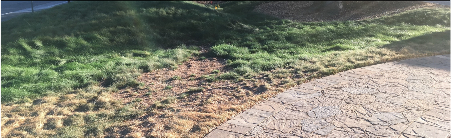
This bioinfiltration system infiltrates runoff from the new central energy facility and parking lot at Stanford University
