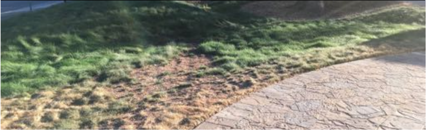
This bioinfiltration system infiltrates runoff from the new central energy facility and parking lot at Stanford University
