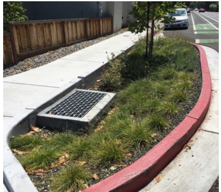
Green infrastructure in Brisbane and the City of Burlingame for neighborhood-scale stormwater capture and diversion (Left: City of Brisbane, Above: Matthew Fabry)
