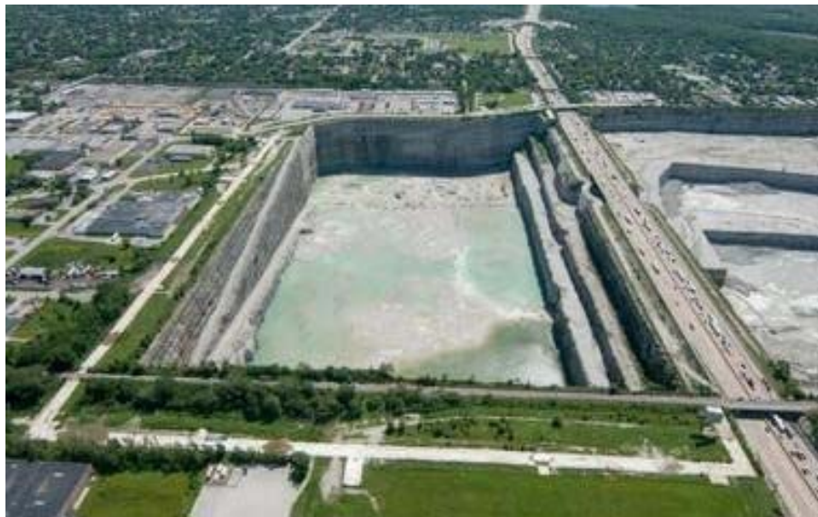
Figure 2-2. Centralizing urban stormwater capture systems usually requires large storage basins, like the City of Chicago's 25,000 AF basin. Locating a similarly sized basin in California would be challenging, and it would sit empty for the long dry season.
