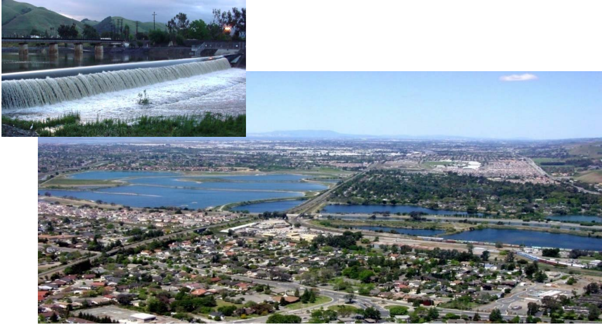
Figure 3-1. ACWD diverts rainfall runoff into former quarry pits for groundwater recharge. Once urban blight, these rehabilitated quarries are now the centerpiece of the Quarry Lakes Regional Recreation Area.
