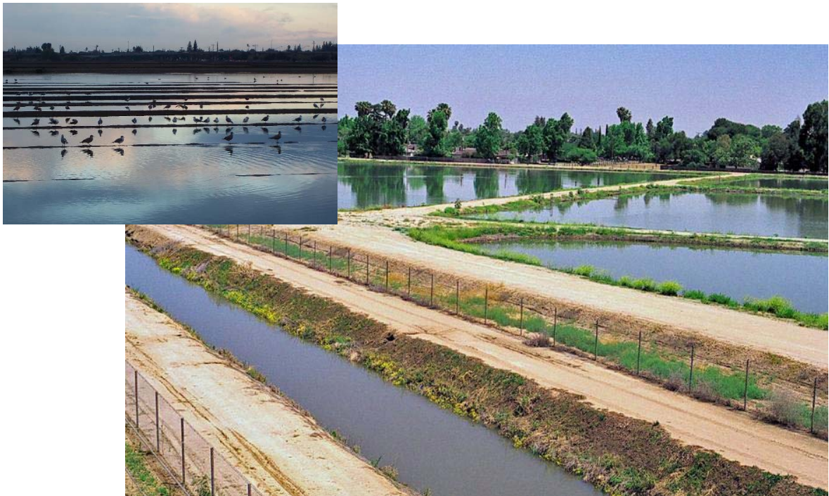
Figure 3-2. Leaky Acres, built in 1970 by the City of Fresno, comprises 26 percolation ponds covering 225 acres, collecting stormwater for groundwater recharge.
