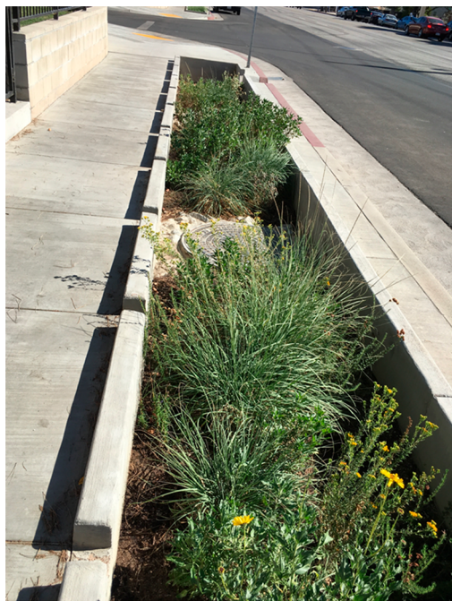
Figure 2. Curbside dry well installation with vegetation in Los Angeles. The system comprises three chambers—one for particle settling with the second and third chambers allowing percolation from the base into crushed rock or by an overflow pipe in the third chamber set into crushed rock. (photo by the authors).
